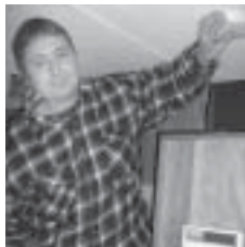
Marshall Worley installs a smoke alarm.
