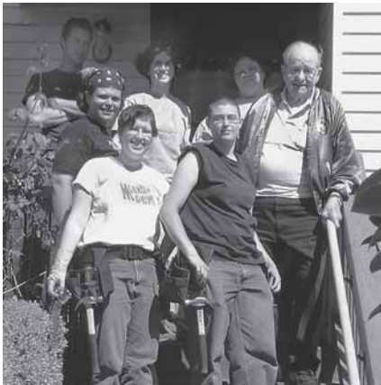
Students from Oregon Tradewomen, Inc. installed railings for Mr. Halverson (right) a Portsmouth neighborhood resident.
