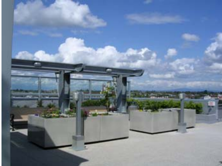
Rooftop drains into tank
